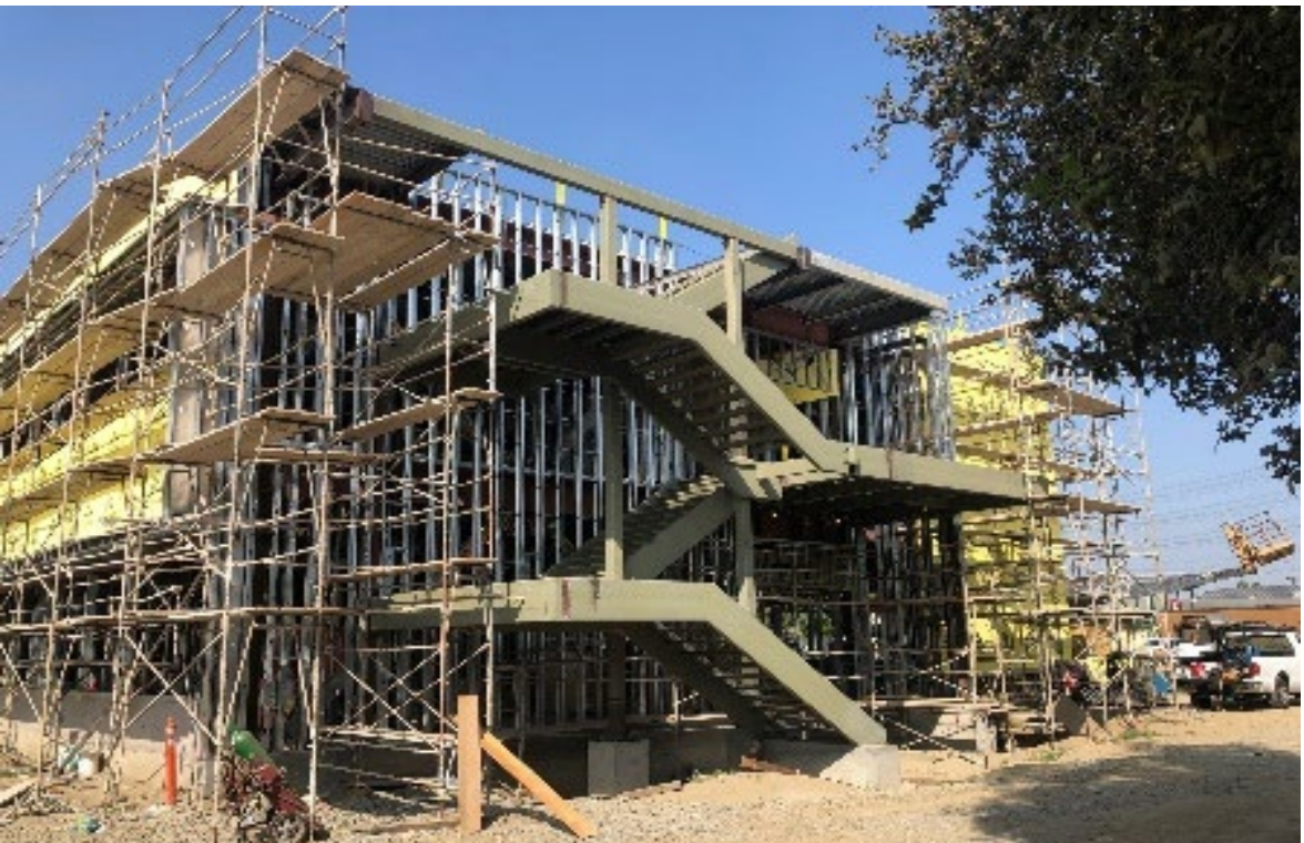
IB #1 Exterior – East Side
