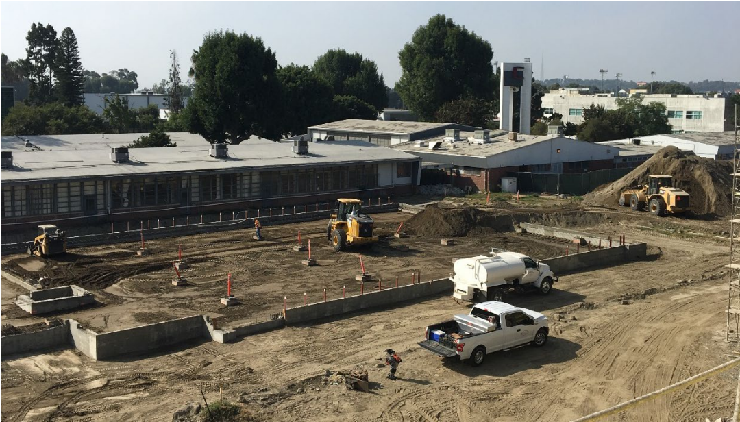
IB #2 Site grading & concrete work
