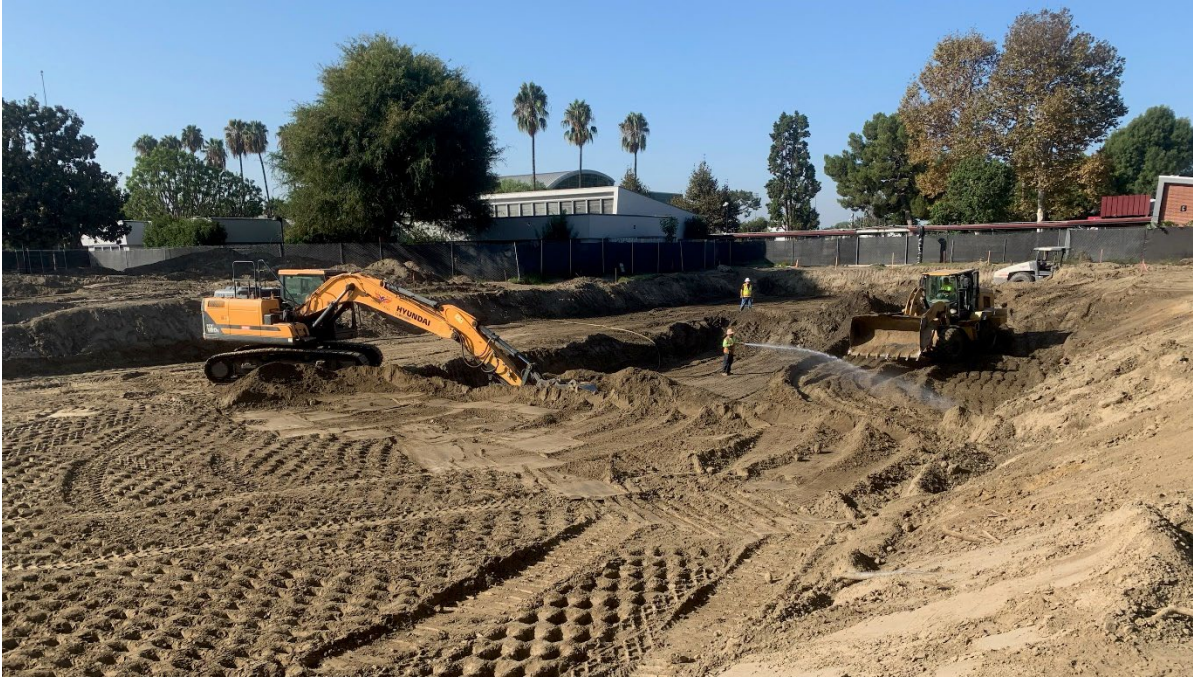
Student Services Building Over Excavation
