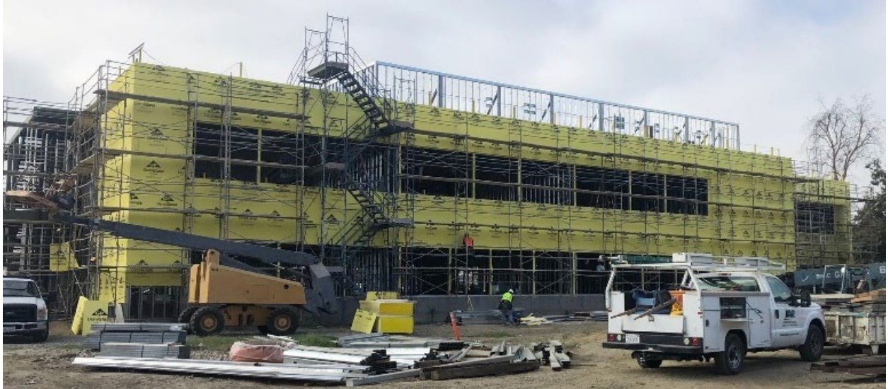
IB #1 Exterior – north side
