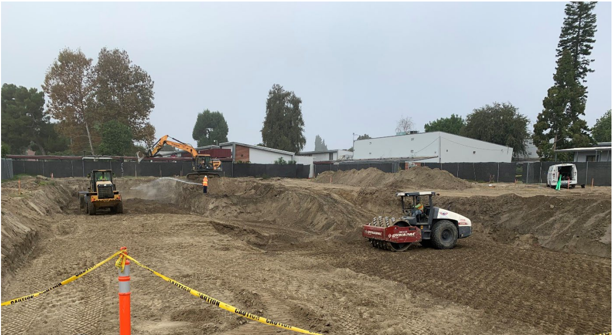
Student Services Building Over Excavation
