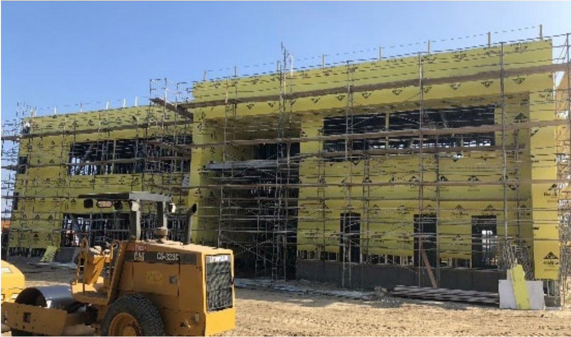
IB #1 Exterior – west side
