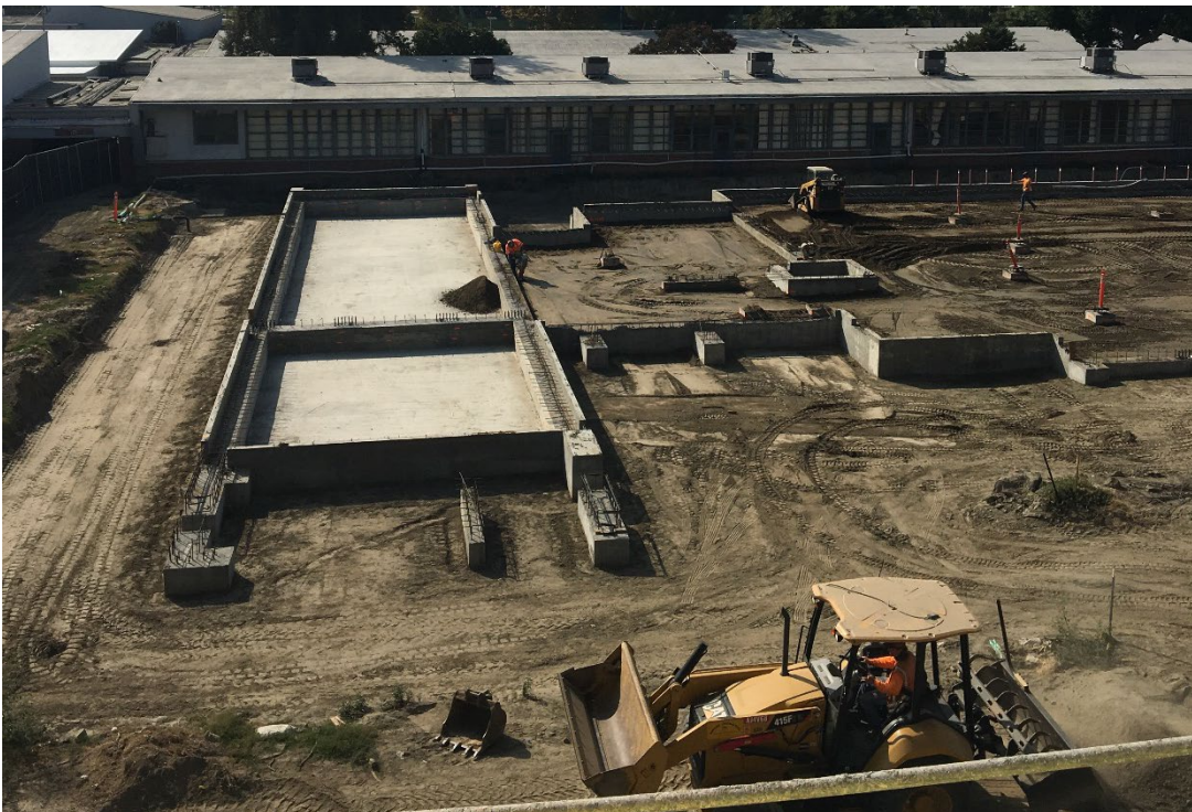
IB #2 Site grading & concrete work
