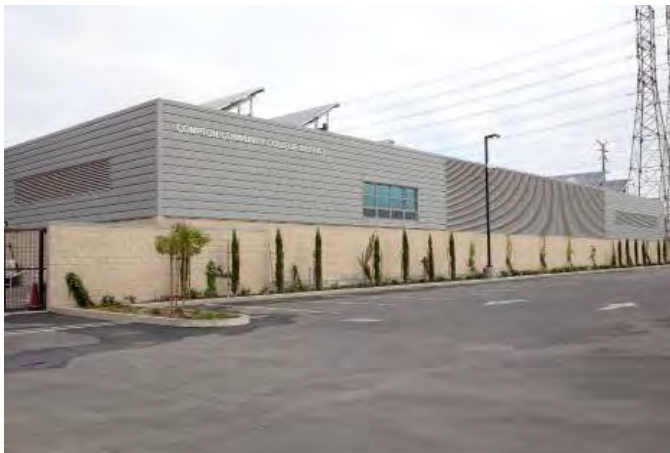
Central Plant and Campus Utility Infrastructure
