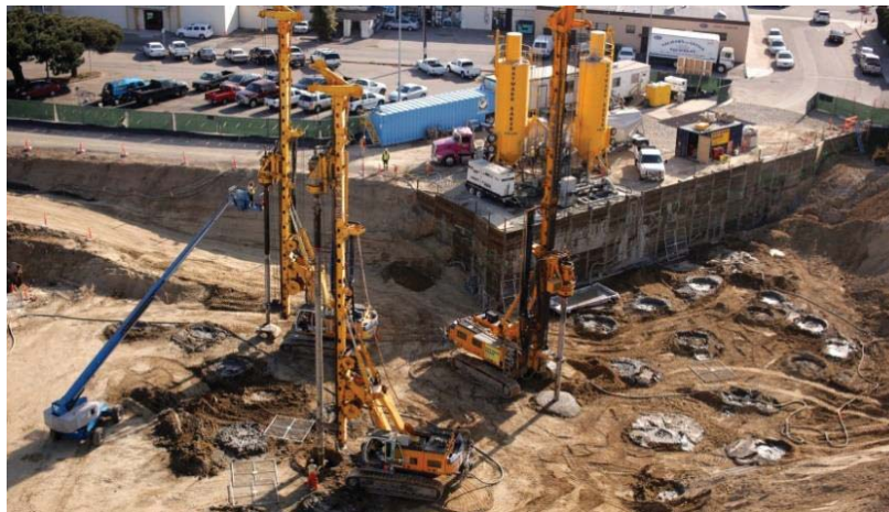
Figure 1: Construction of DSM
