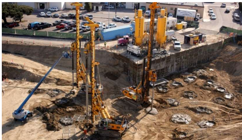
Figure 1: Construction of DSM
