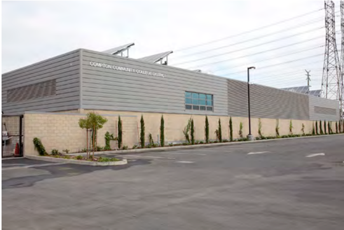
Central Plant and Campus Utility Infrastructure
