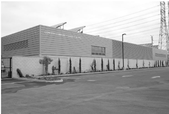
Central Plant and Campus Utility Infrastructure
