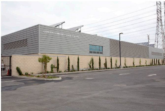
Central Plant and Campus Utility Infrastructure
