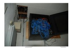
In most of the offices and classroom computer laboratories the cable is exposed and in some cases run over floors where it is subject to damage by foot traffic.
